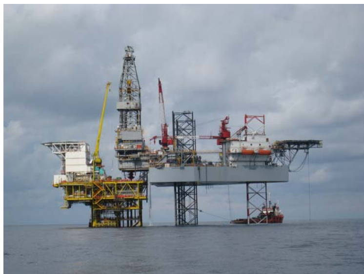
The E. Belumut "A" platform which recently commenced production.
